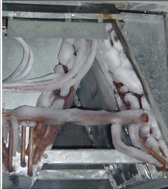
ICED EVAPORATOR COILS
